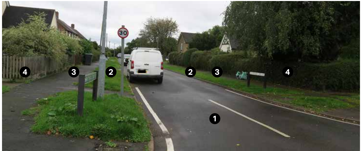
Figure 37: Downer Drive, a tertiary road framed by green verges planted hedges. It is recommended that footways along the street are minimum 2m wide and that parking is provided in the form of inset bays to avoid impeding traffic.
