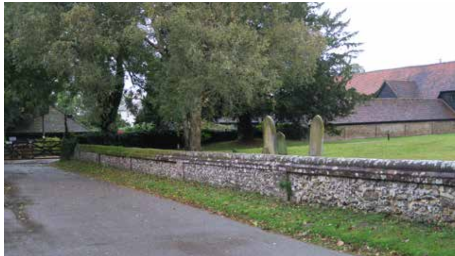
Figure 72: Church yard wall built with local flint.
