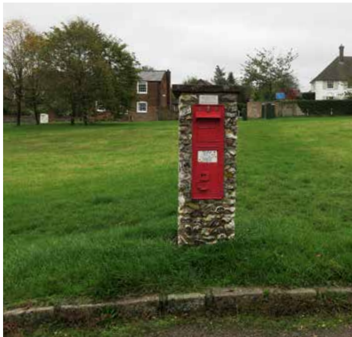
Figure 81: Red letter box encased in masonry.
