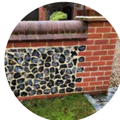
Knapped flint and red brick boundary wall
