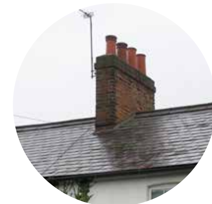
Red brick chimney
