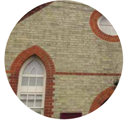
Red brick trim and yellow brick infilling
