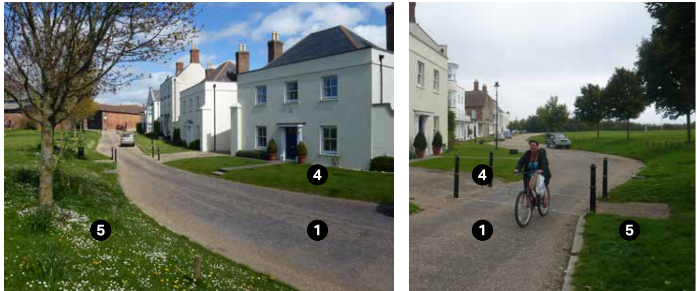
Figure 42: Examples of edge lanes in Dorchester, with low-speed roads shared between motor vehicles and cyclists, and opportunities for on-street parking (note: some localities may prefer clearly defined footways and parking bays).
