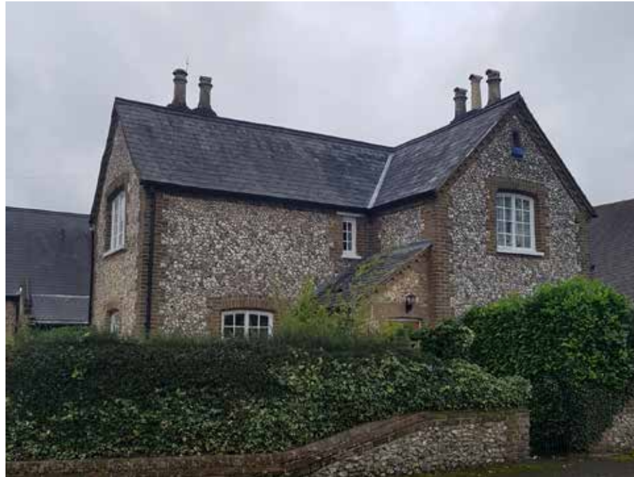
Figure 71: Buildings exhibiting a use of traditional local materials - knapped flint, red brick, slate, and clay plain tiles.
