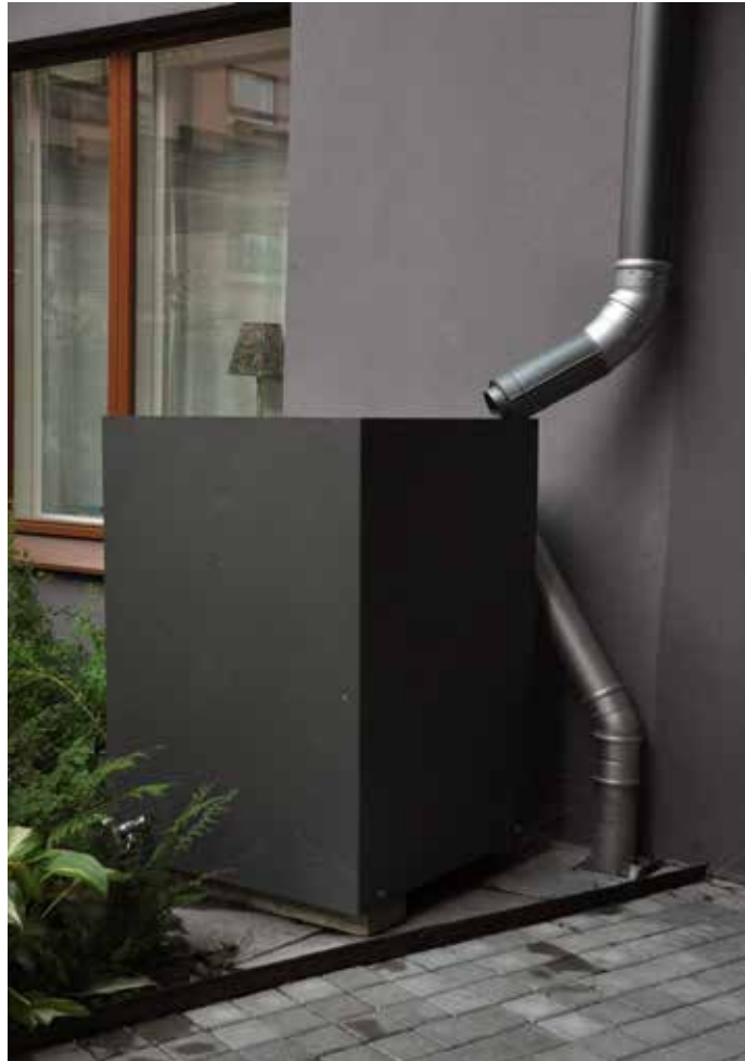
Figure 87: Examples of tanks used for rainwater harvesting.
