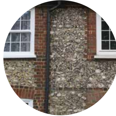
Red brick trim and knapped flint infilling
