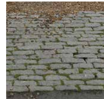
Granite block vehicle crossover
