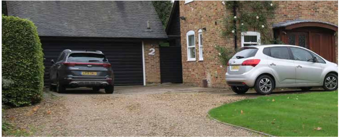
Figure 55: Side garage (left) designed as a secondary mass to the main residential building and built with a matching material palette.
