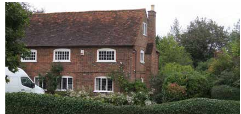
Green End Farmhouse - red brick façade with upper floor horizontal sliding sash windows and ground floor multi-pane casement windows with cambered heads.
