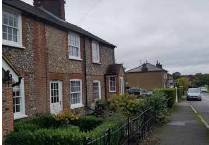
Figure 6: Red brick and knapped flint building with red brick decoration to accentuate details.
