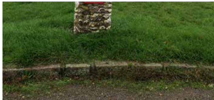
Figure 78: Granite kerbs along the Green.
