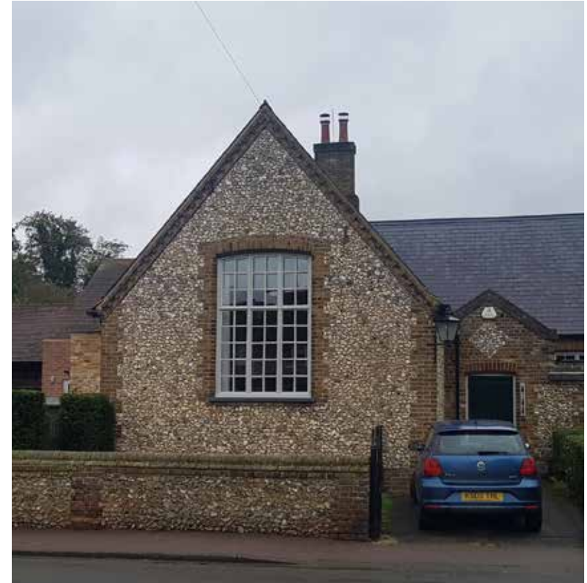
Quoins and window trims in yellow stock brick with knapped flint infilling. Detailed brickwork highlighting eaves and house entrance. Boundary wall with matching materials.
