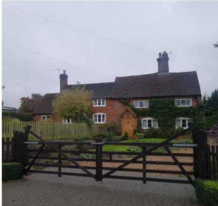
Figure 11: Red brick building with clay plaintile roof.
